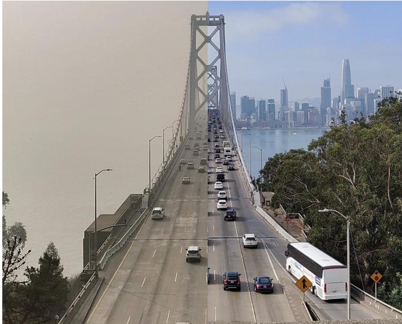
Bay Bridge, 170 miles from Paradise, CA
