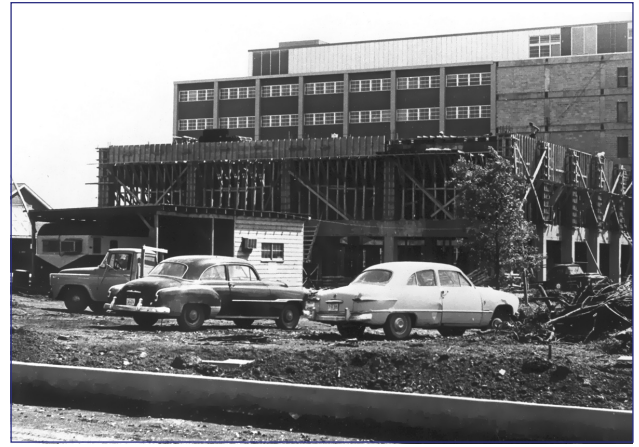
The A.B. Chandler Medical Center under construction ca. 1960
